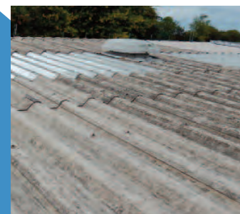
Cleaned Roof Surface
