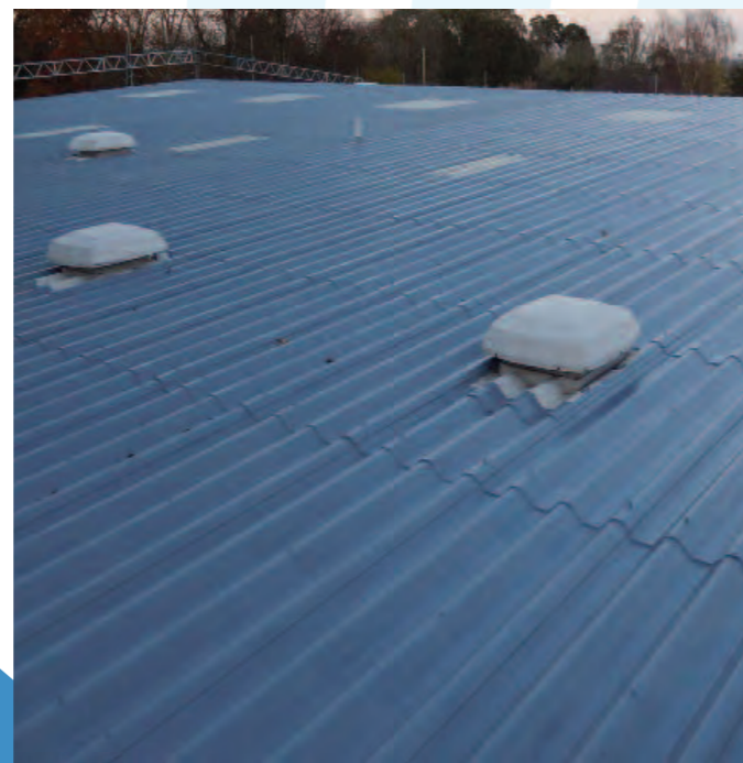
Asbestoseal 20 to entire Roof
