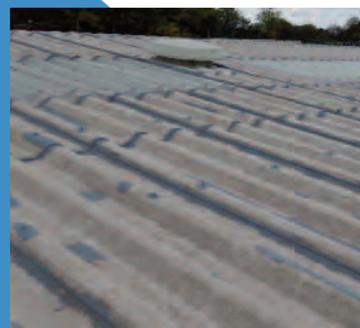
Liquasil Non-Sag Sealer to Overlaps and Cracks
